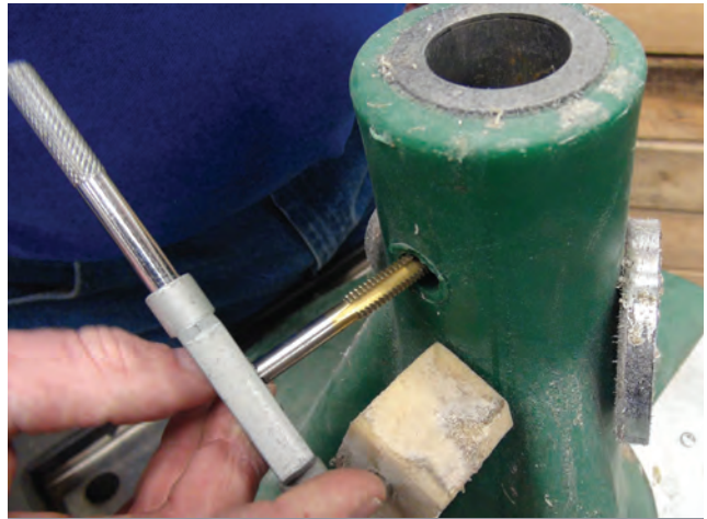
RUN A 3/8"-16 TAP THROUGH THE OPENING OF THE TENSION KNOB NUT – A SINGLE TIME SHOULD BE ENOUGH.
